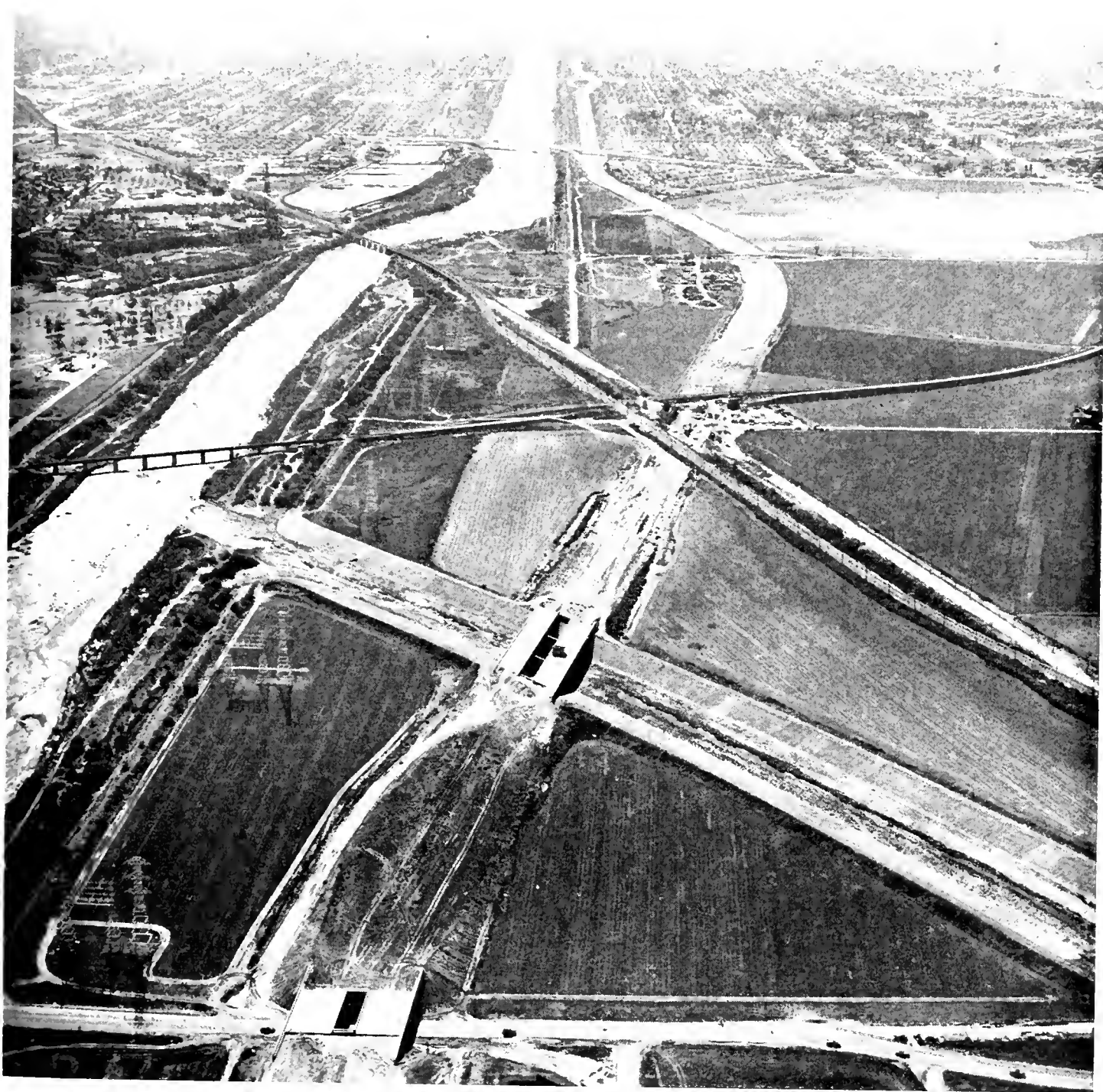
Aerial view looking southerly along the Lang Beach Freeway, showing Los Angeles River on left, Del Ama Bridge in foreground, Campton Creek Bridge next, and the railroad grade separation bridges with Pacific Electric Railway and Union Pacific Railroad at Dominguez Street in center of photograph. In background is completed portion of Lang Beach Freeway in use by public from Willow Street to Anaheim Street in City of Long Beach. Long Beach harbor in background.
